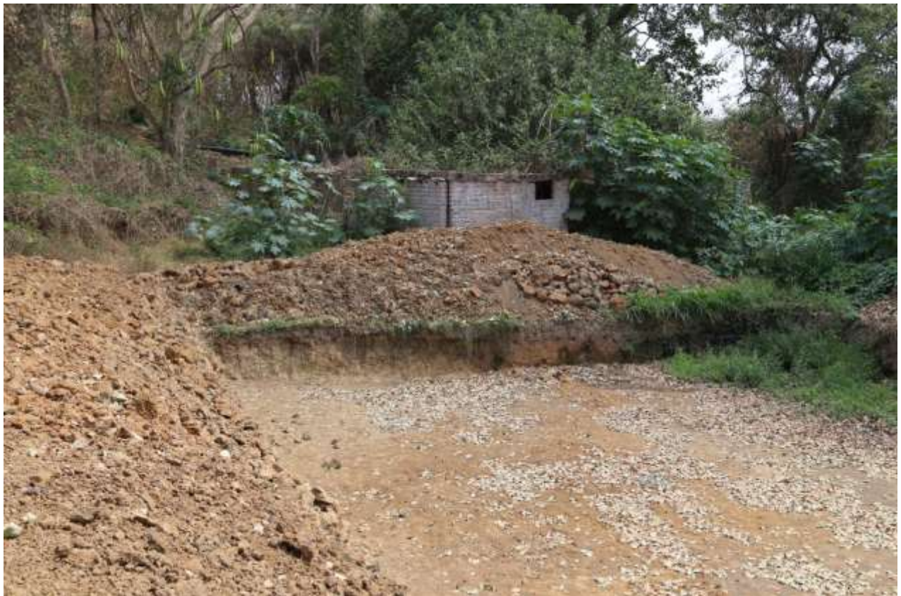
Dig: Reed sewage treatment plant, In the background: Septictank 90 000 l
