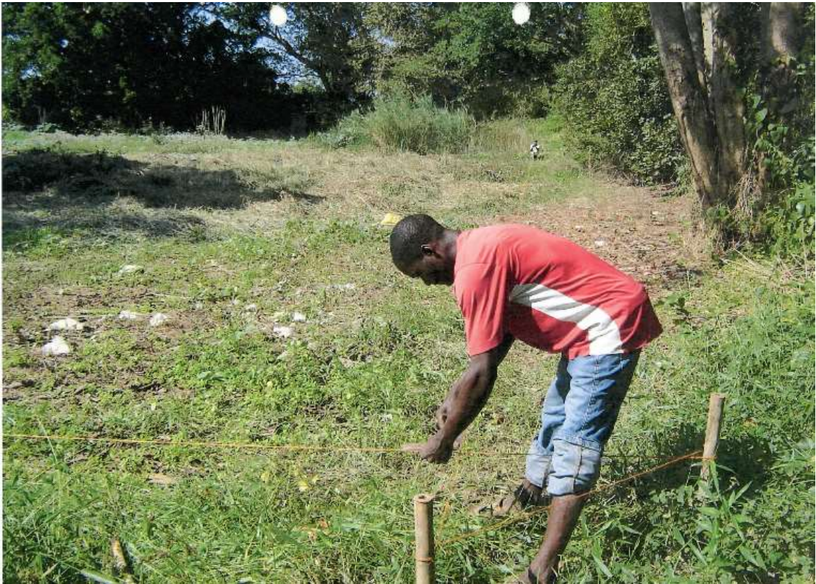
Reference line reed sewage treatment plant
